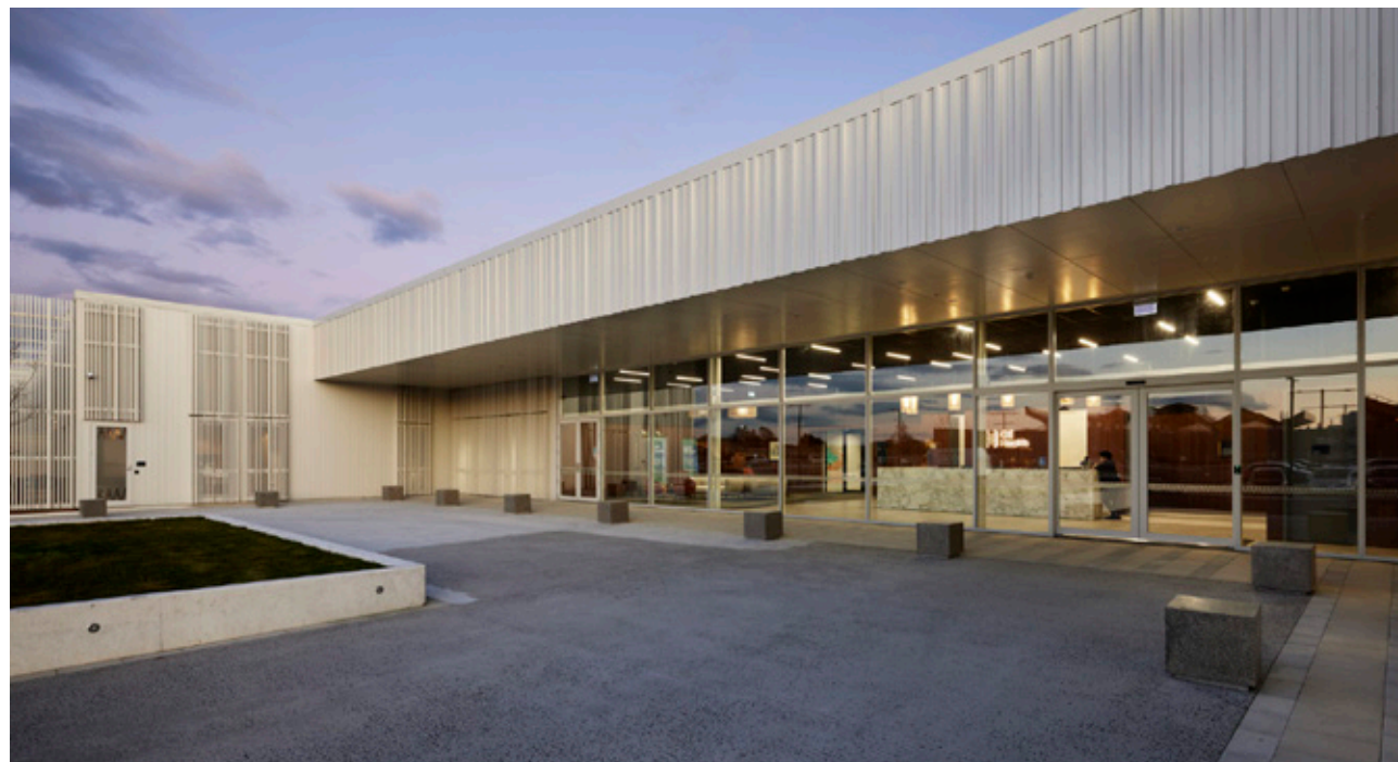
QE Health Rebuild – centre for clinical health and wellness Rotorua, Bay of Plenty
